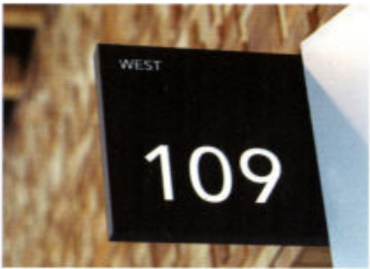
Narrow-profile acrylic sheets and room number signs use low-energy LEDs for illumination.
