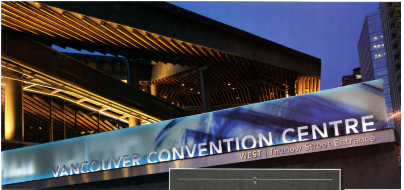
The 31,665-m 2 West Building opened in 2009, in time to host the International Broadcast Centre for the 2010 Winter Olympics.
